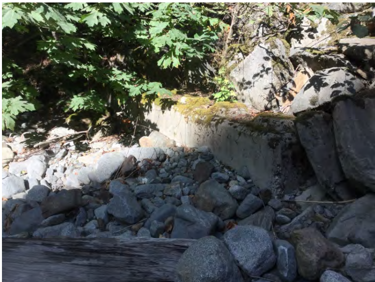
Lock blocks downstream right bank
