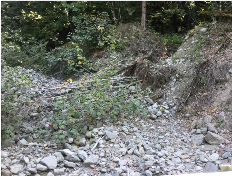
Debris in channel upstream
