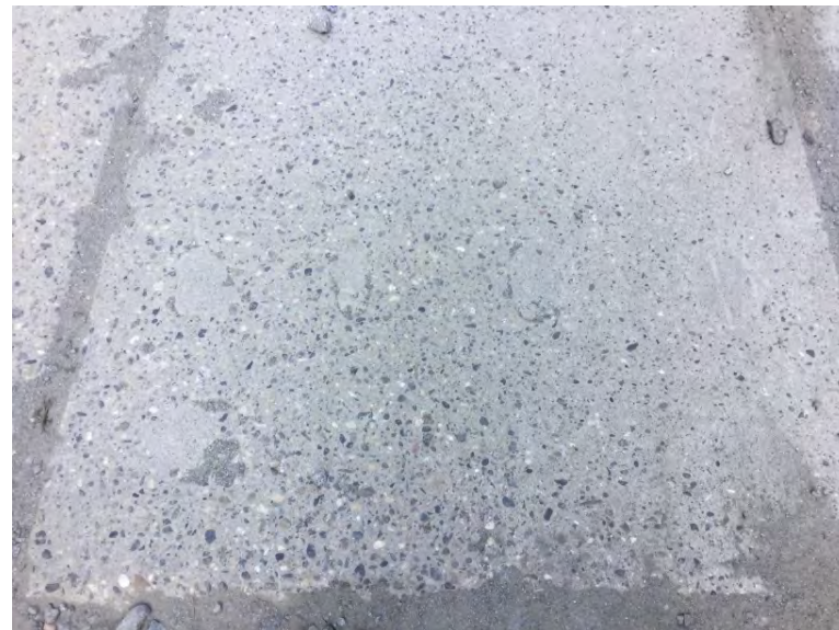
Each slab appears to have 4 connections at abutment
