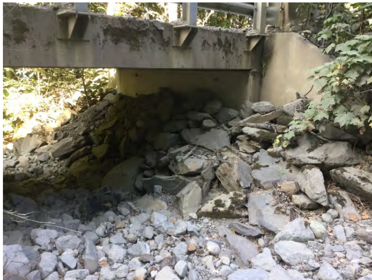
Right Bank Abutment when facing downstream
