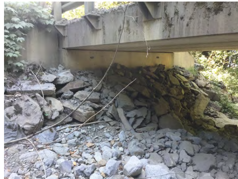
Left Bank Abutment when facing downstream
